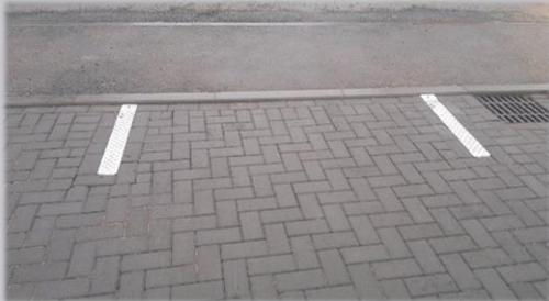
When not in use, our SB11BP post tucks neatly into a coffin type box which is concreted into the ground, giving it a completely flush surface, allowing you to drive over it to your hearts content. Ideal where you have block paving and need a good post to fit neatly in. Completed with an integral lock (comes with two keys) and also available keyed alike for quantities of two or more at an extra cost. Our SB11BP is coated with a Zinc Plated finish to protect against the weather and rusting.
